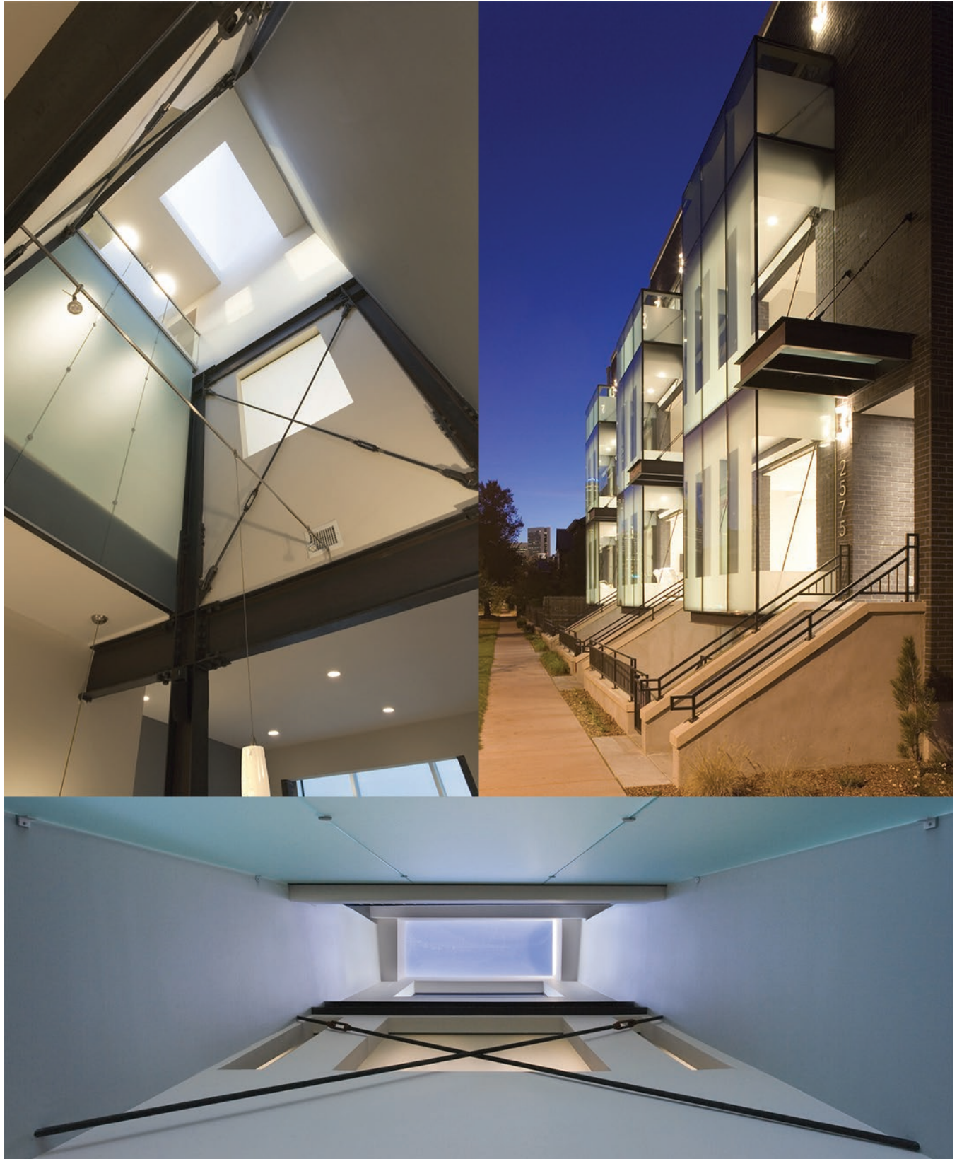
Figure 4. Merchants Row Brownstones - glass bays - three story light wells, in situ Design.
